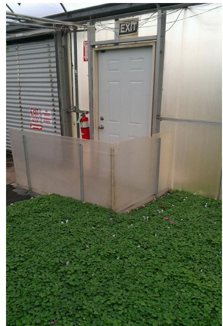
Figure 3. A polycarbonate barrier has been used in this greenhouse to prevent cold air from lowering the plant temperature of crops near the door.
