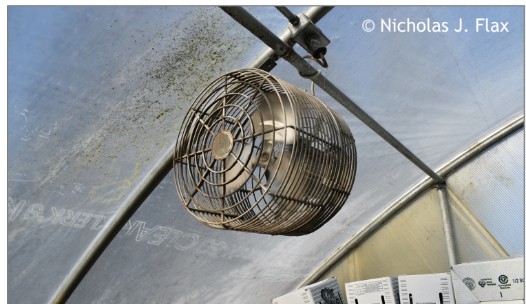
Fig. 4. Increasing airflow in your production environment is an effective way to reduce powdery mildew pressure. Whether the number of horizontal air flow (HAF) fans or total air movement is increased, both are meaningful steps to reduce disease.
