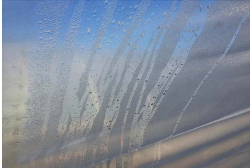
This image was taken at 3:00 pm! Condensate happens, yes, but proper ventilation and irrigation should minimize its presence.
